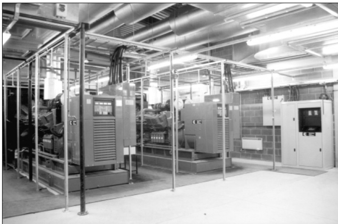
Twin 800 DFHD sets (1000 kVA) with QST30 G4 engines, PCC control and DMC autosync cubicle in a typical installation.
